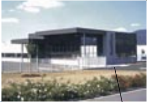
Kutting France S.A.R.L. Niederbronn-Les-Bains, France
