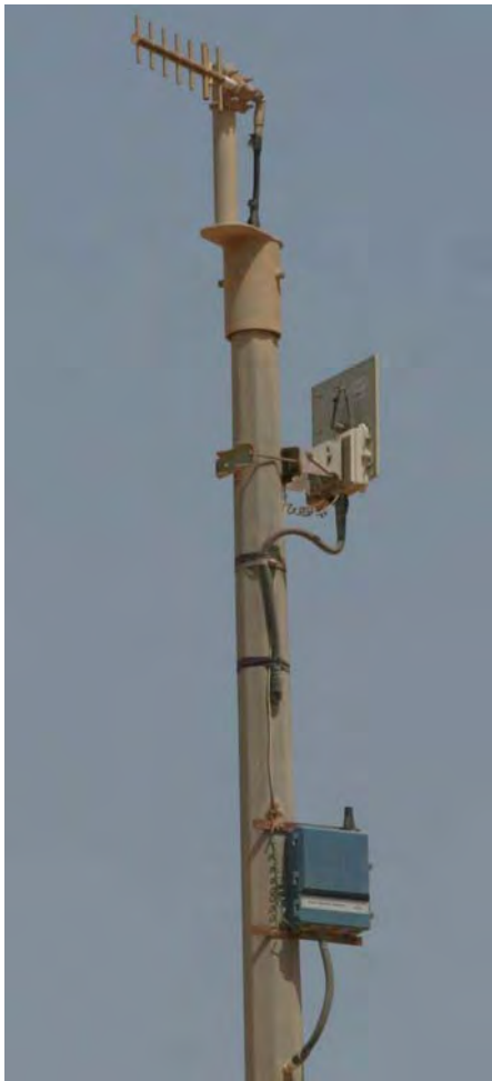
Fig. 5. Personnel and tracking applications need a plantwide Wi-Fi coverage for tracking RFID tags, often accomplished by external aerial mounting of wireless transmitters and receivers.
