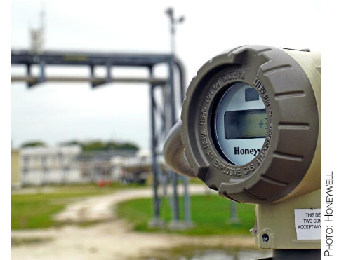
Wireless sender for ISA100.11a: It can operate with an update rate of 1s, but at the expense of battery life.
